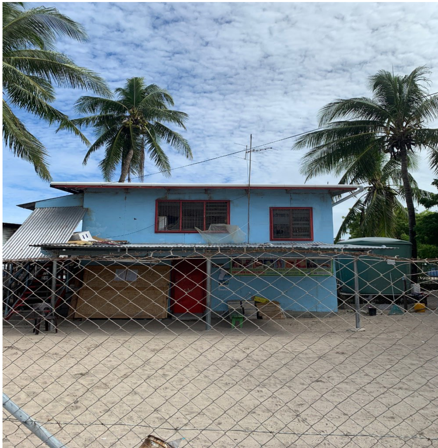
Plate 1. Porebada Sub Health Centre in 2019
