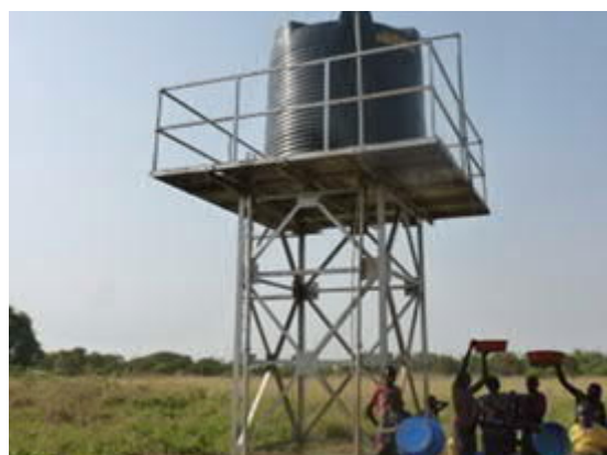
Solar Water Tower, Ngwedo TC
