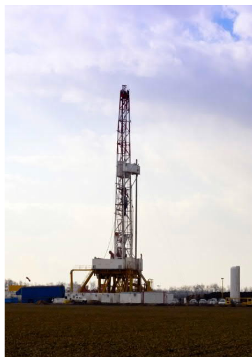
Typical Drilling Rig
