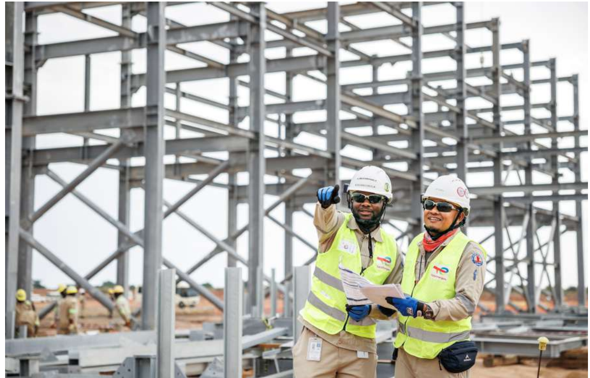
Pipe rack construction at Central Processing Facility
