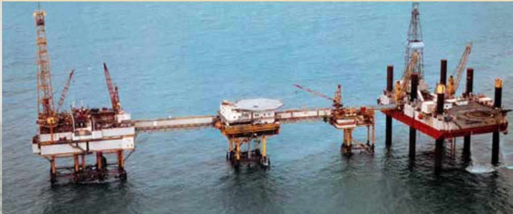
In order to maintain gas production, a fourth platform, the L7-PK compression platform, was installed in 1981 alongside L7-CC.
