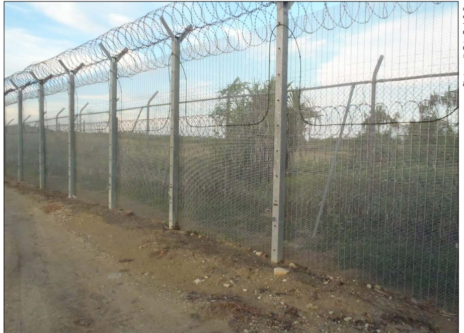
Plate 2.8 LNG Plant security fence (close up)
