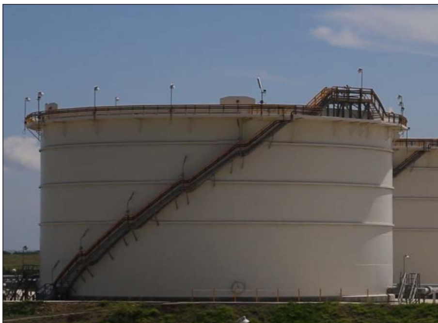
Plate 2.6 Naphtha storage tanks
