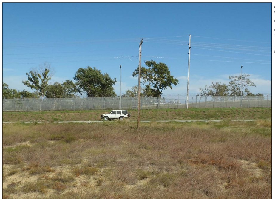
Plate 2.9 LNG Plant security fence and bypass road
