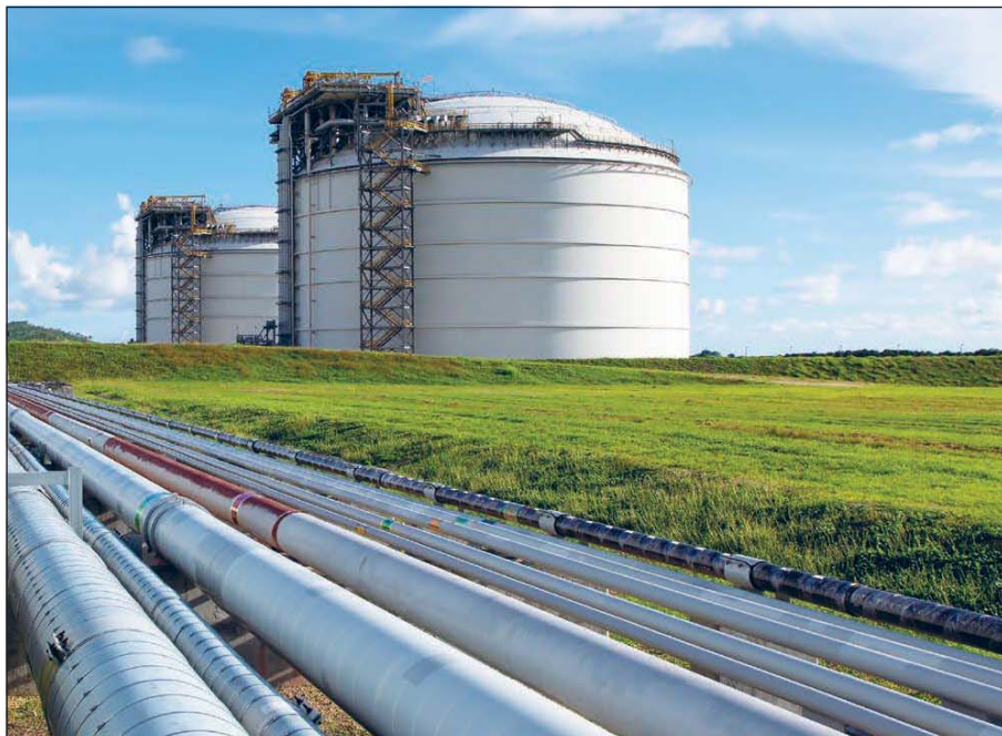
Plate 2.4 LNG storage tanks and connecting pipework
