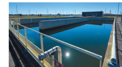
Collection basin for rainwater from the Bayet natural gas combined cycle power plant
