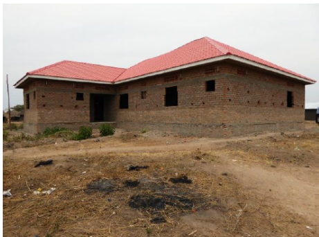
Brick house in construction (for a Taxi Operator), Masaka
