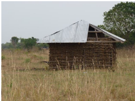
Iron-roof house in construction, Bugana-Kichoke
