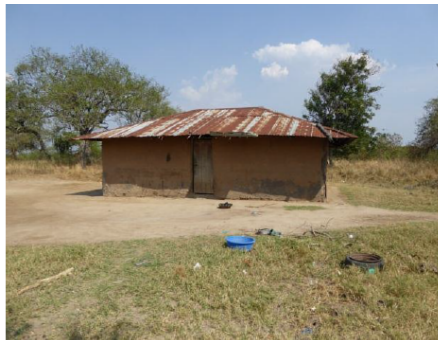
Iron-roof house, Kijangi
