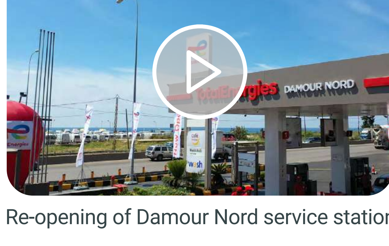
Re-opening of Damour Nord service station
