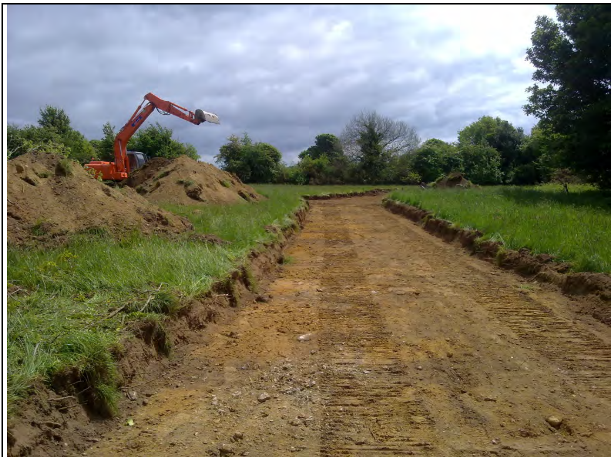
Figure 2.4-3 Typical Topsoil Removal
