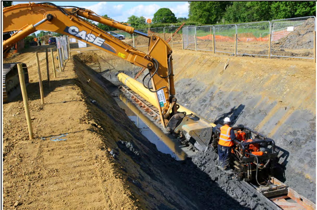
Figure 2.4-15 Auger Bore
