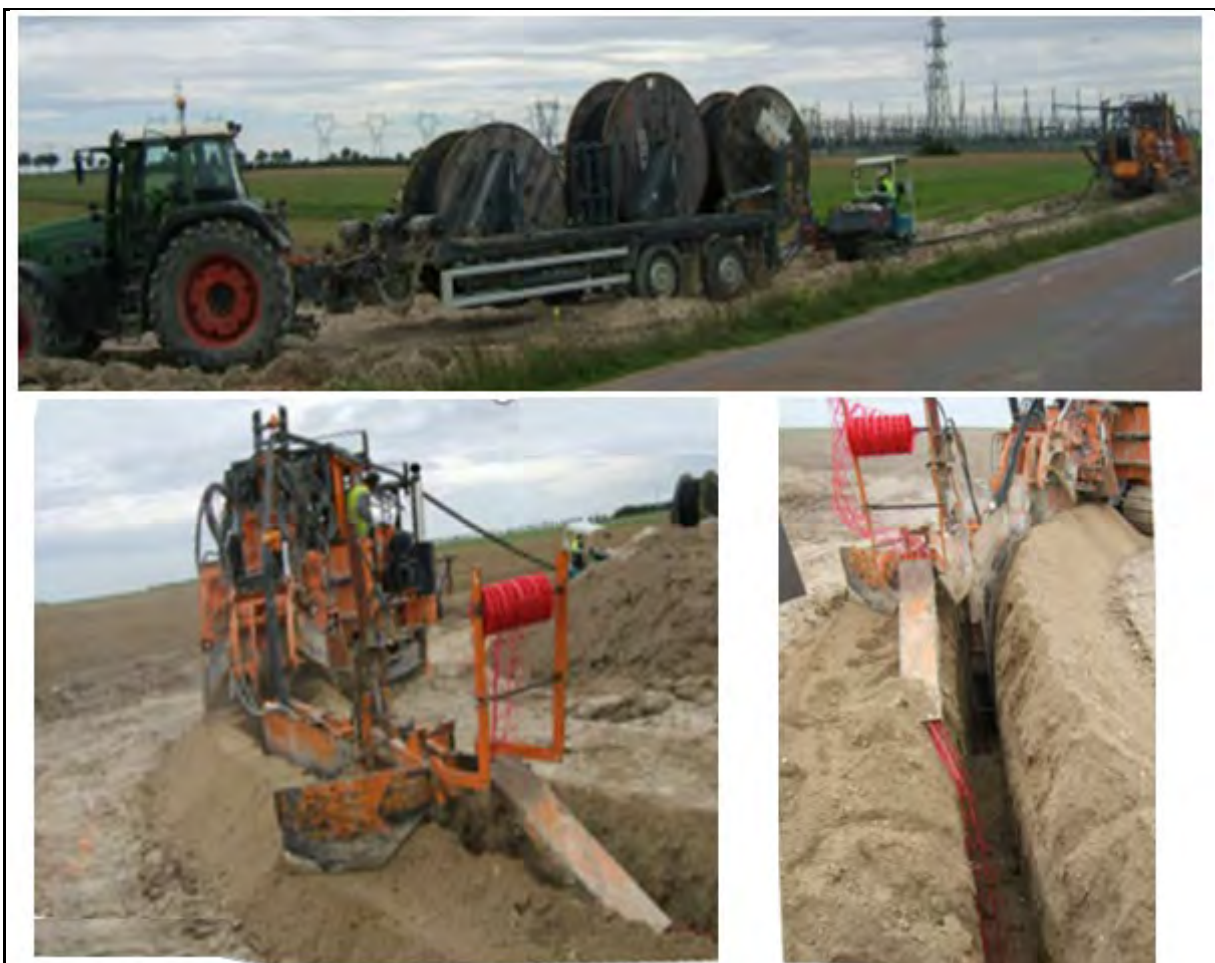
Figure 2.4-11 High Voltage Power Cable Installation
