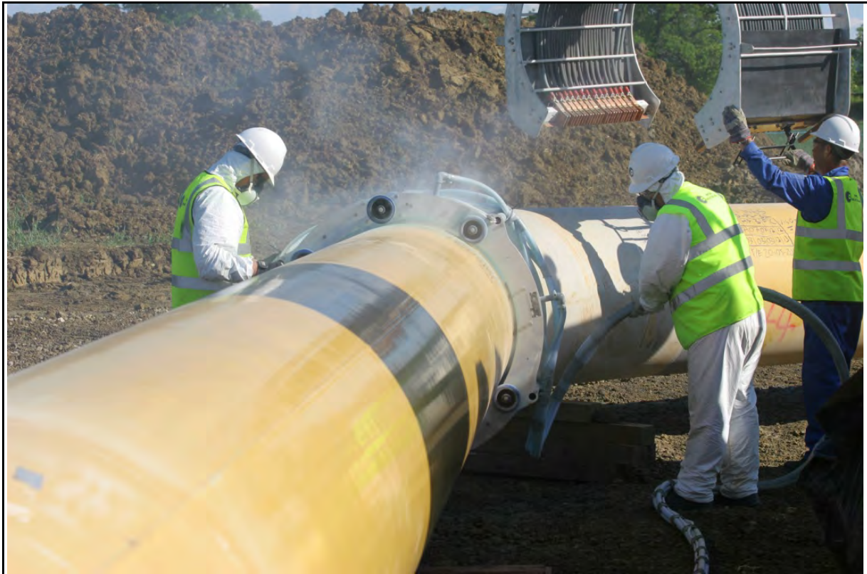
Figure 2.4-8 Anti-Corrosion Field Joint Coating
