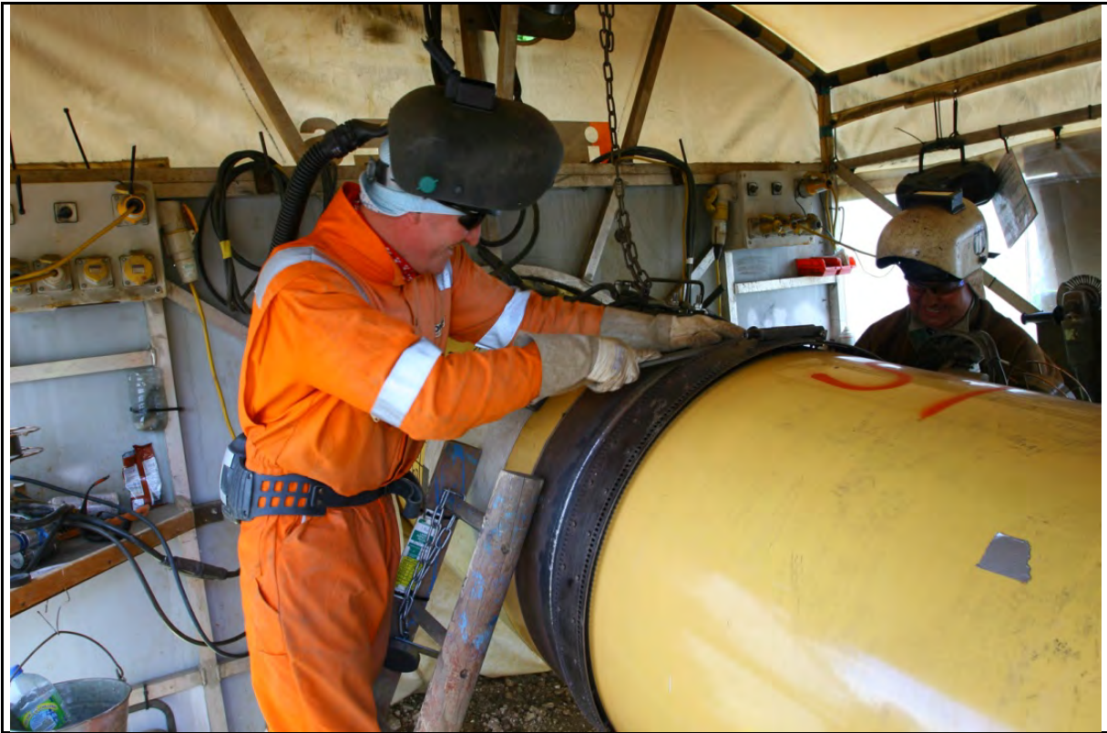
Figure 2.4-6 Typical Pipeline Welding
