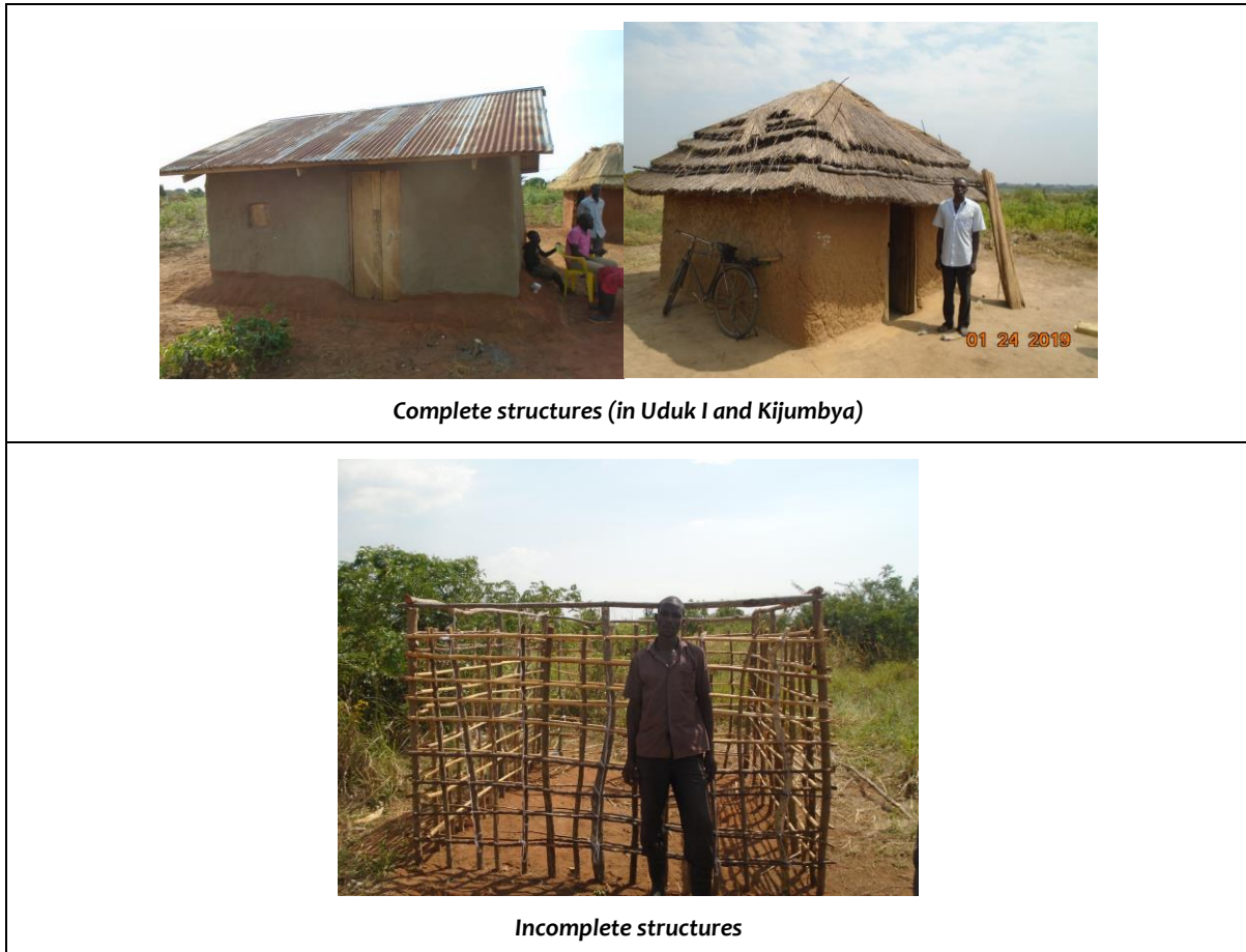
Figure 8.3: Sample structures in the RAP 3b project area
