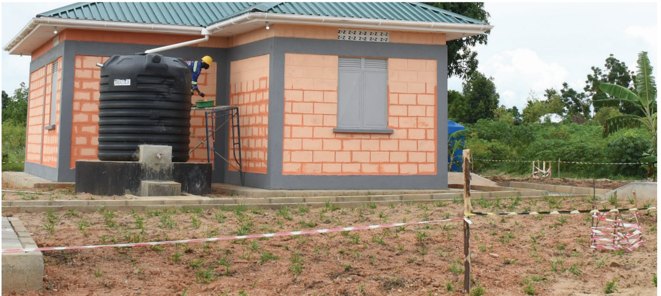
Okecha's house in Avogera in Ngwedo Sub-county, Bullisa district ready for occupation.
