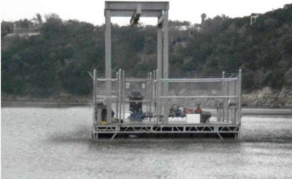
Figure 4-10: Example of an Offshore Fixed Floating Platform
