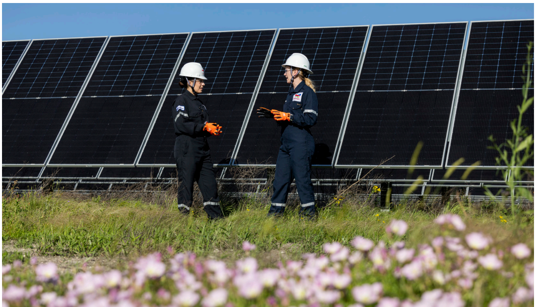
Danish Fields, TotalEnergies' largest solar farm in the United States, features 1.4 million ground-mounted photovoltaic panels.
