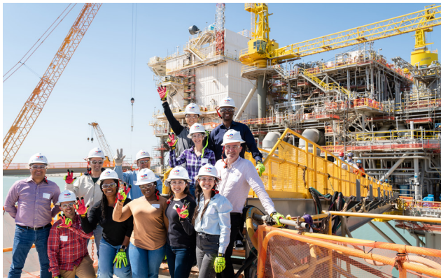
The TotalEnergies' team visits the Anchor platform before it sails away to the U.S. Gulf Coast.
