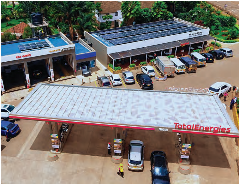
Solar panels installed at our service station
