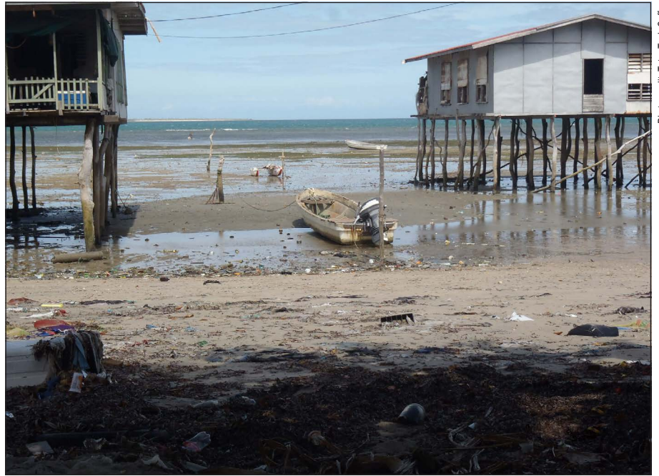
Plate 5.1 Fishing vessels next to houses built using mangrove posts
