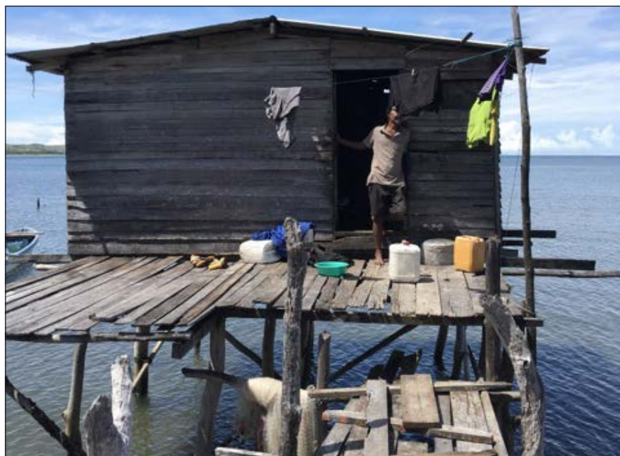
Plate 5.6 Wooden house with mangrove posts elevated over water in Boera
