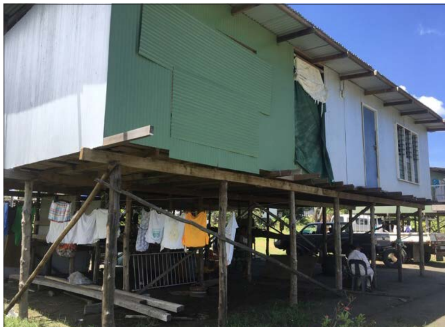
Plate 5.4 House with kapa sheeting and mangrove posts in Lea Lea
