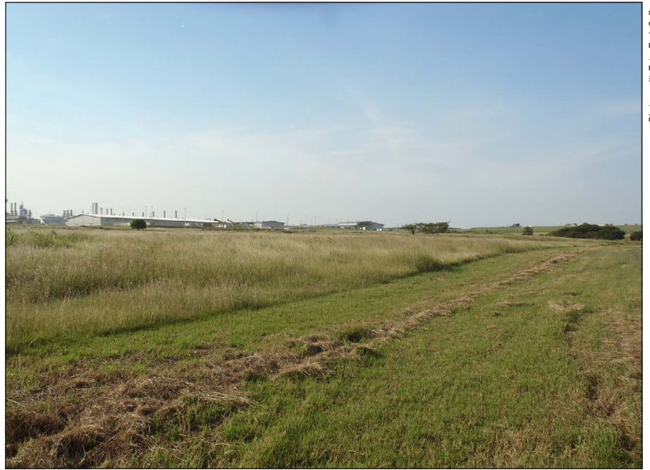
Plate 7.1 LNG Plant site facilities looking north-east
